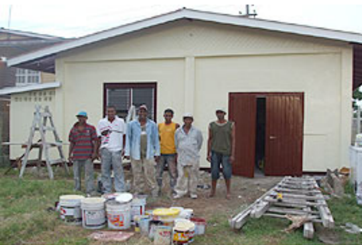
Almost Completed Building
