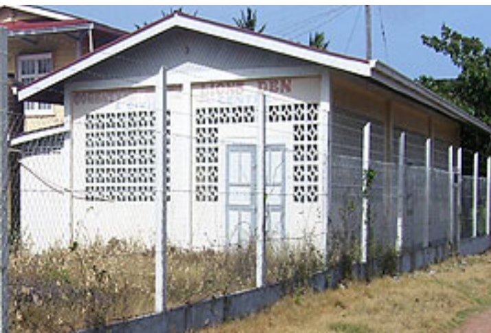
Lions Club before Renovation
